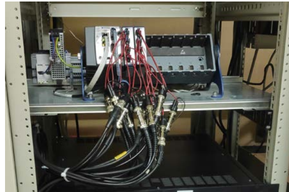
Setup of the vibration acquisition on site
