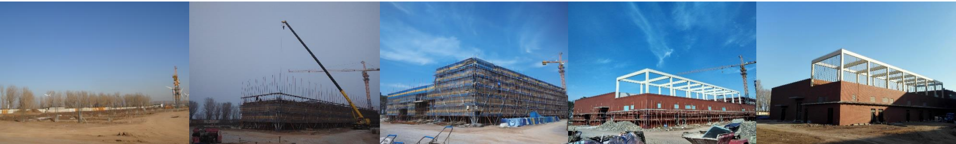
2014.11- 2016.01 DCLS Building construction
