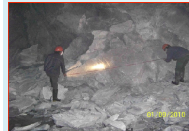
Rockburst of 6.3m³ during dig
