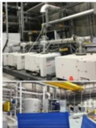
Compressors and Oil Removal System (WCS)
