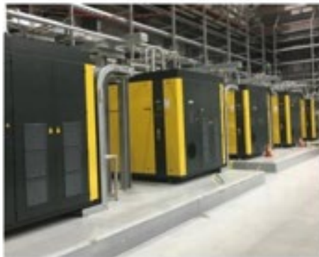
Compressors and Oil Removal System (WCS)
