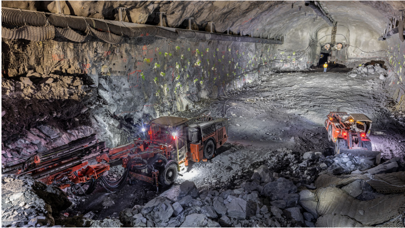
Excavation of caverns for DUNE Far Detector
