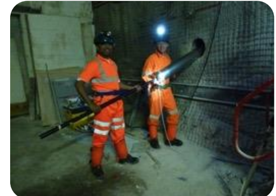
Bore hole detector installation
